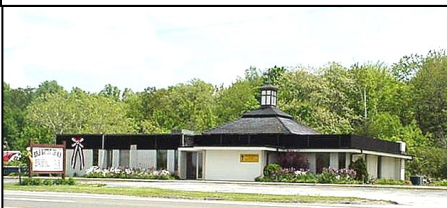
One of the buildings that the Richfield Bible Baptist Church utilized for many years. Now used by a local business.
