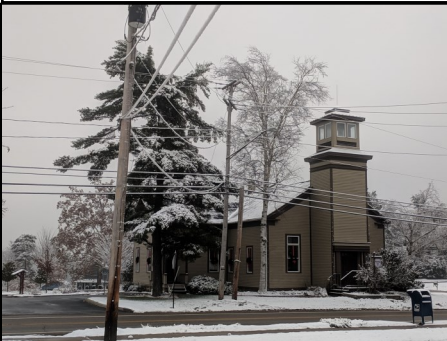
The first Richfield Baptist Church building. Now the known as the Fellowship Hall.
